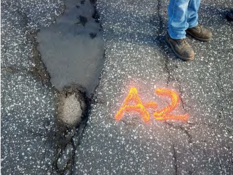
Figure 3.2 Pothole A-2 prior to Patching (After Cleaning).
