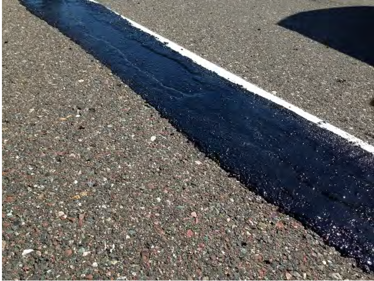
Figure 3.54 Finished Mastic Patch.
