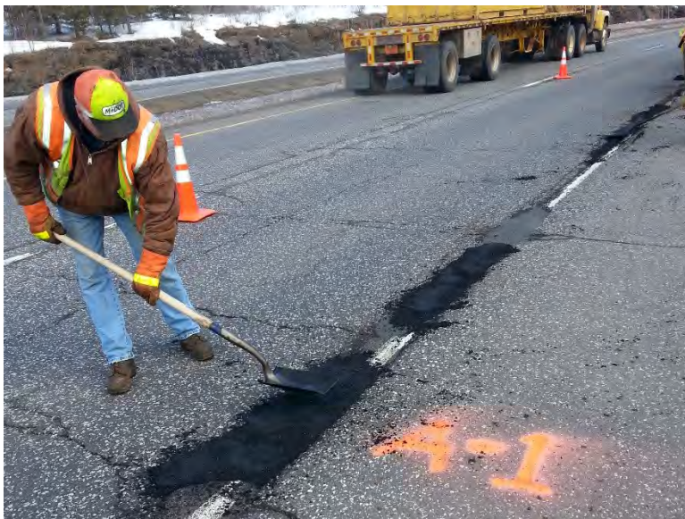
Figure 3.6 Pothole A-1 after Patching.
