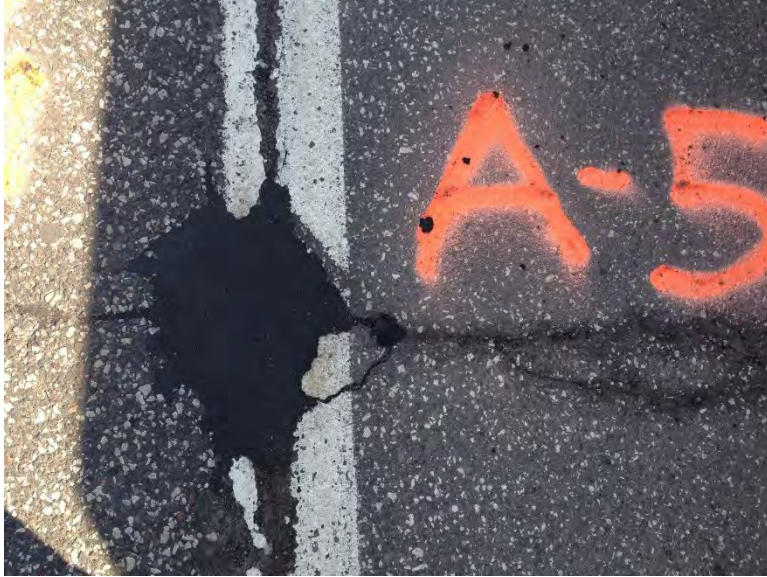
Figure 3.17 Pothole A-5 (3 Days after Patching).
