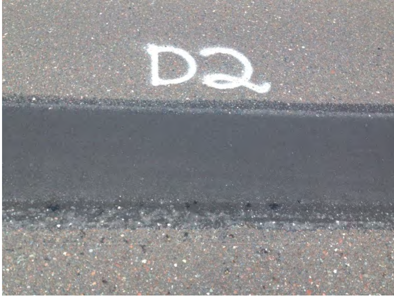
Figure 3.64 Pothole D-2 (35 Days after Patching).
