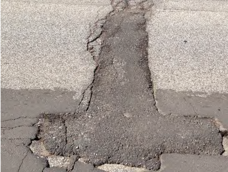
Figure 3.44 Pothole B-5 (146 Days after Patching).
