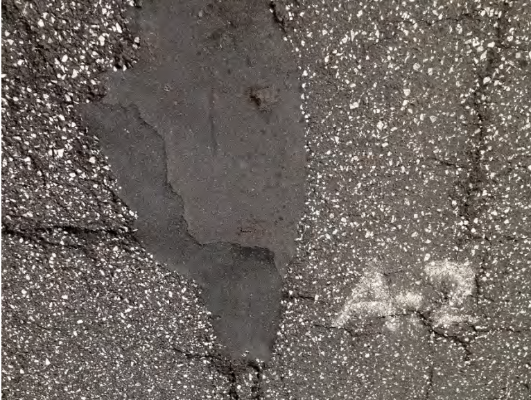
Figure 3.12 Pothole A-2 (149 Days after Patching).
