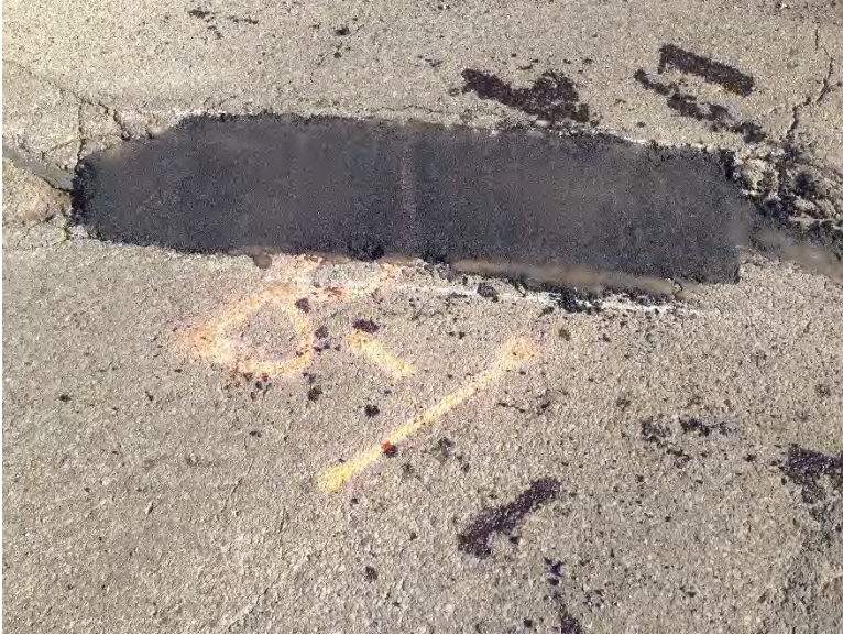
Figure 3.32 Pothole B-1 after Patching.
