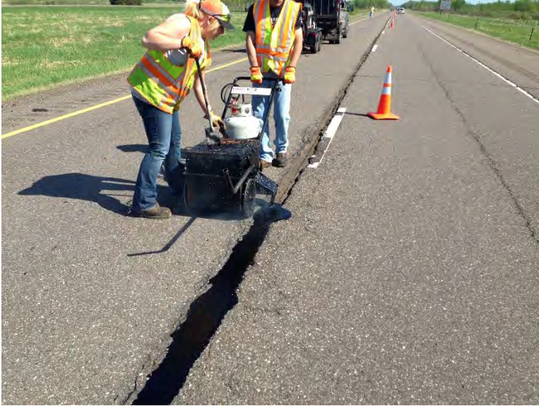
Figure 3.52 Filling Longitudinal Crack with Mastic.
