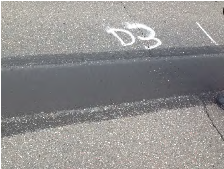
Figure 3.65 Pothole D-3 (35 Days after Patching).
