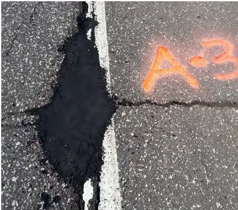
Figure 3.8 Pothole A-3 after Patching.
