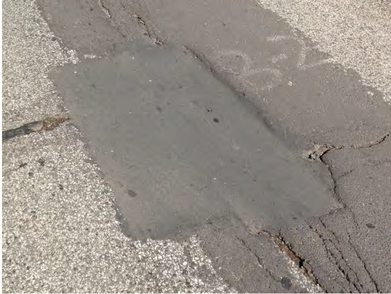
Figure 3.40 Pothole B-5 (146 Days after Patching).
