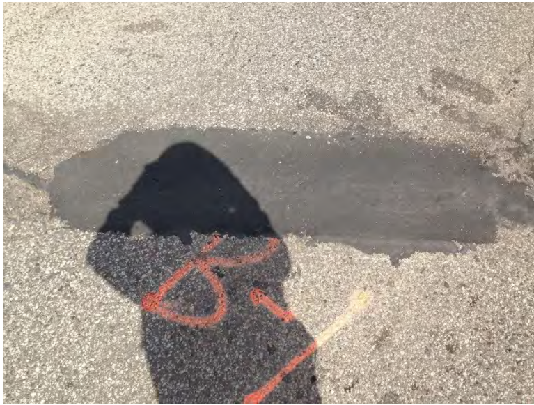
Figure 3.37 Pothole B-1 (3 Days after Patching).
