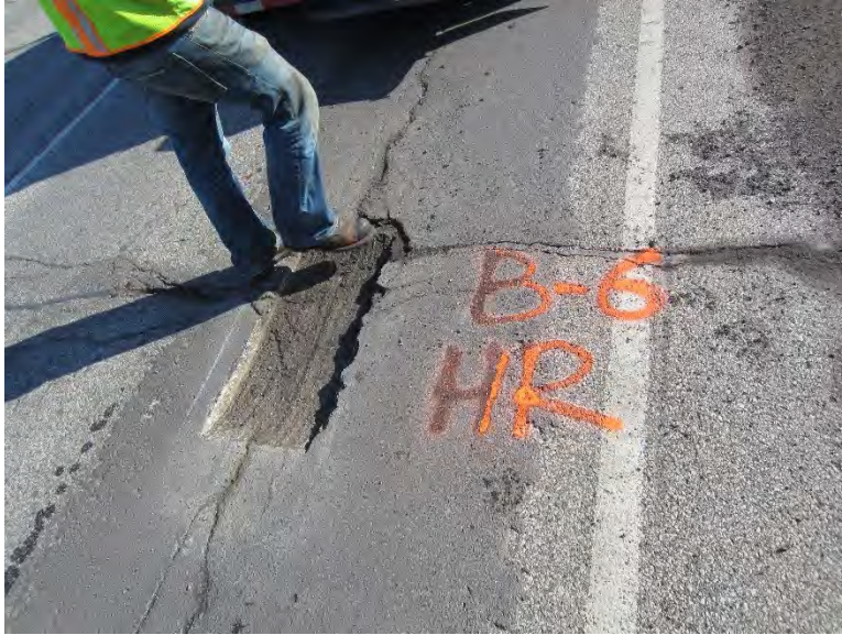
Figure 3.31 Pothole B-6 after Milling.
