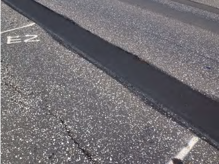
Figure 3.78 Pothole E-2 (28 Days after Patching).
