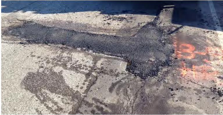
Figure 3.34 Pothole B-5 after Patching.
