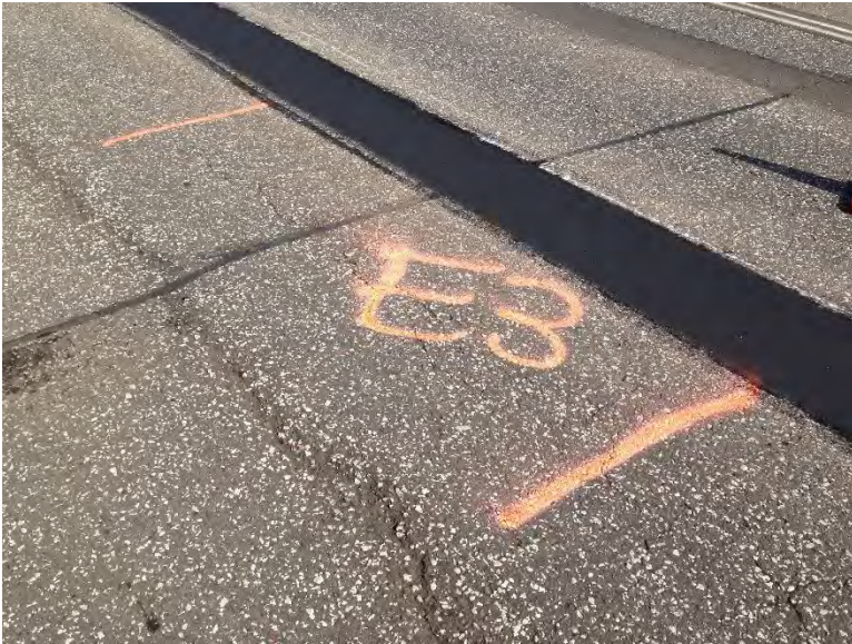
Figure 3.74 Pothole E-3 after Compaction.
