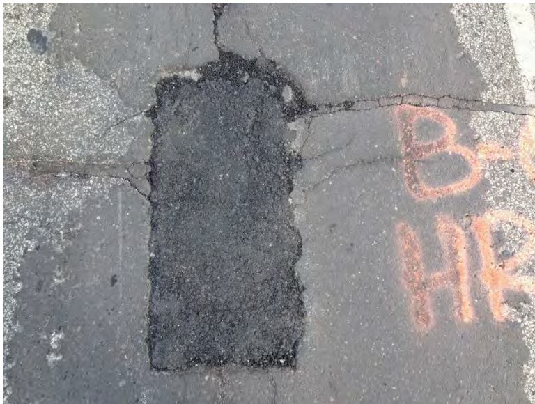
Figure 3.46 Pothole B-6 (3 Days after Patching).
