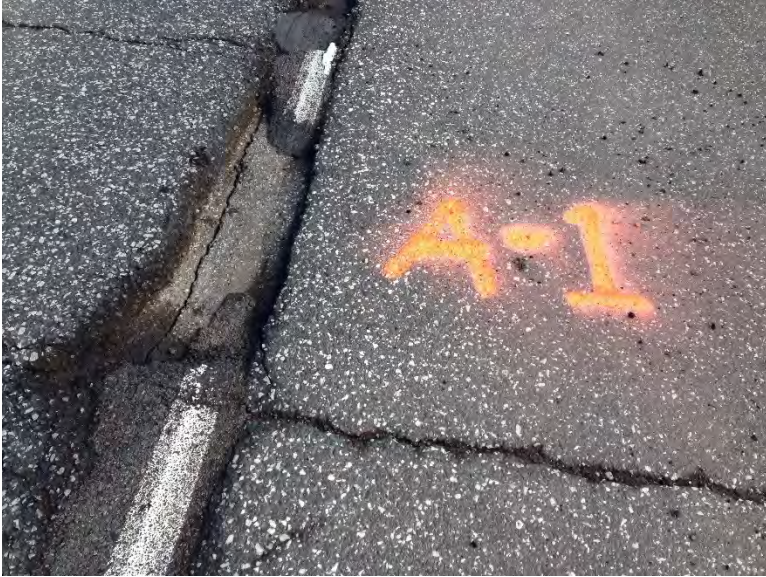
Figure 3.1 Pothole A-1 prior to Patching (After Cleaning).
