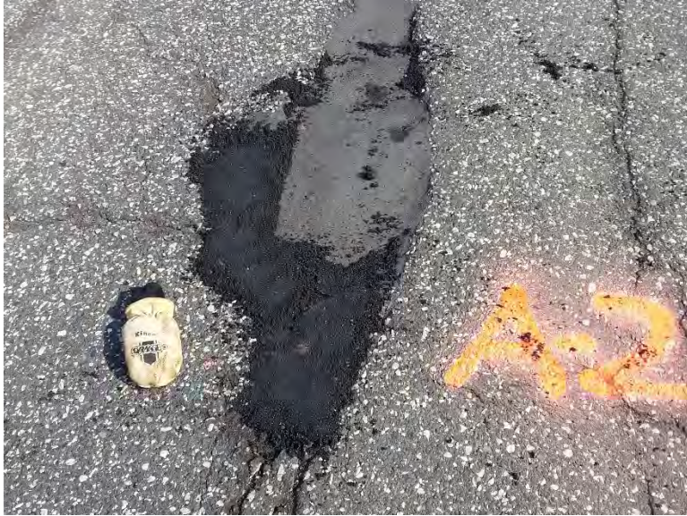
Figure 3.7 Pothole A-2 after Patching.
