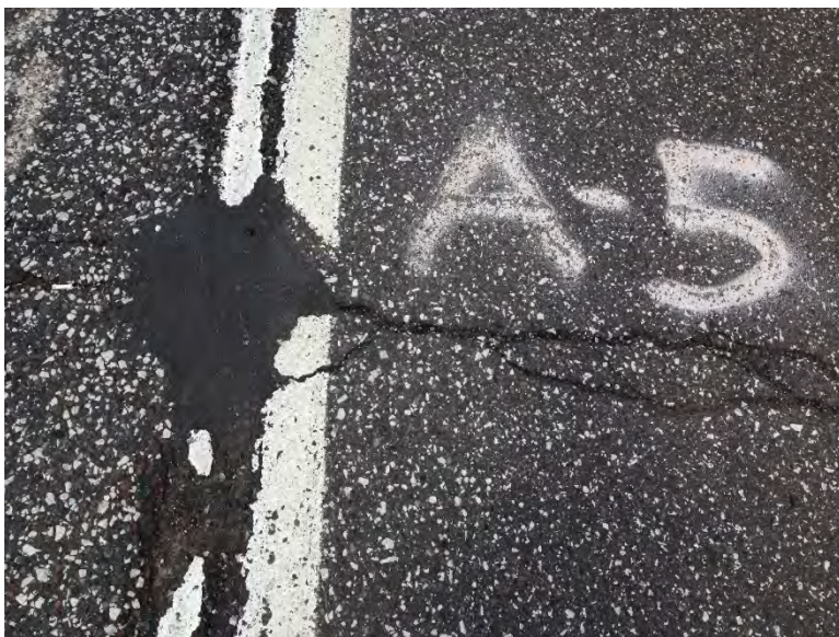
Figure 3.18 Pothole A-5 (92 Days after Patching).
