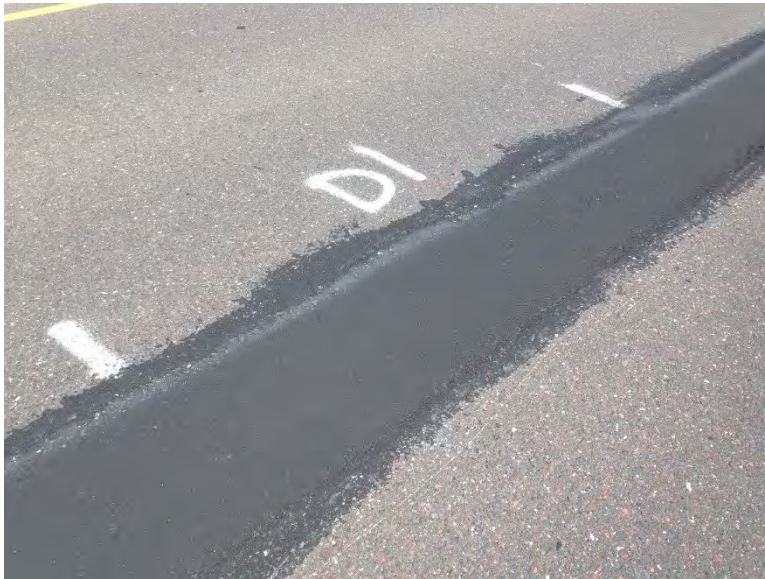
Figure 3.63 Pothole D-1 (35 Days after Patching).
