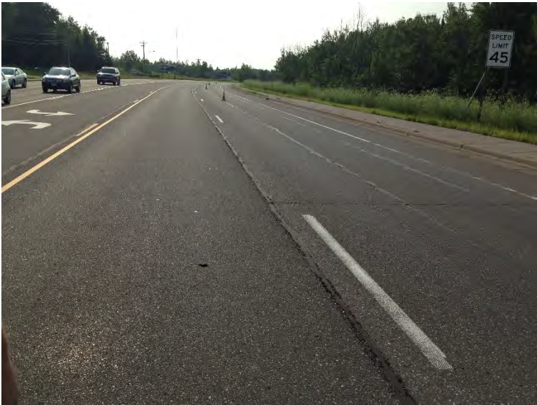
Figure 3.55 Longitudinal Crack along Trinity Road.
