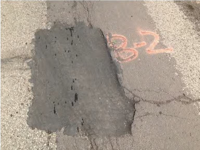
Figure 3.39 Pothole B-2 (3 Days after Patching).
