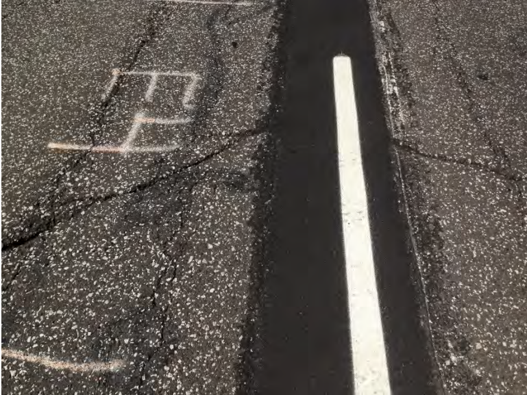
Figure 3.79 Pothole E-4 (28 Days after Patching).
