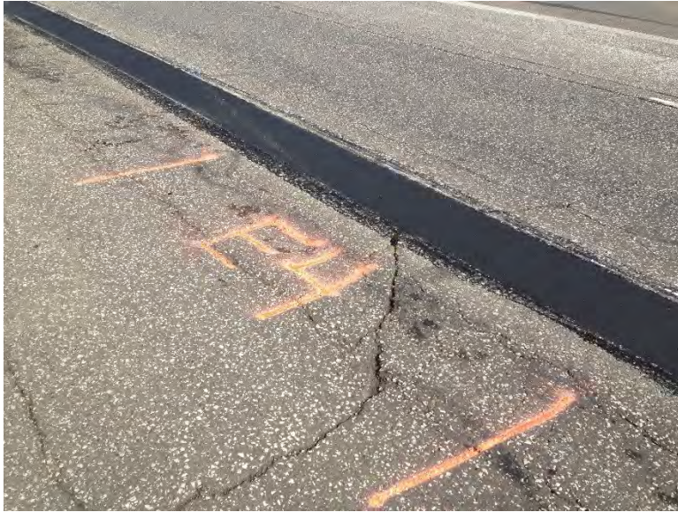
Figure 3.75 Pothole E-4 with Transverse Crack.
