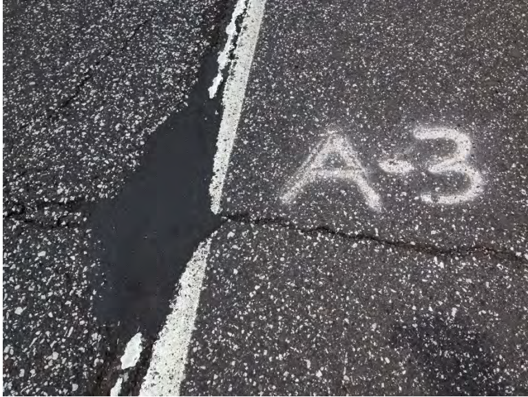
Figure 3.13 Pothole A-3 (149 Days after Patching).
