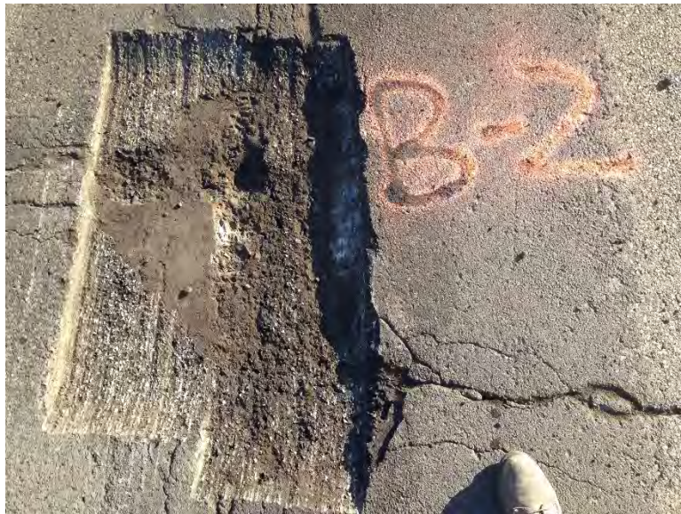
Figure 3.26 Pothole B-2 after Milling.
