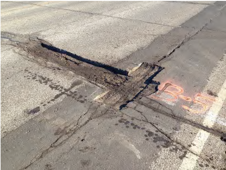
Figure 3.30 Pothole B-5 after Milling.
