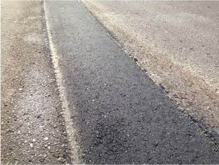
Figure 3.60 Pothole D-2 with Clean Compaction.
