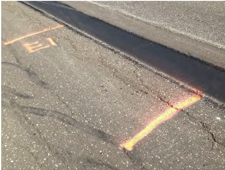
Figure 3.72 Pothole E-1 with Parallel Longitudinal Cracking.
