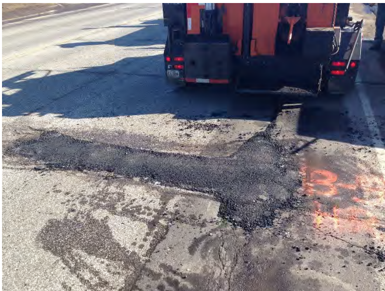
Figure 3.42 Pothole B-5 after Patching.
