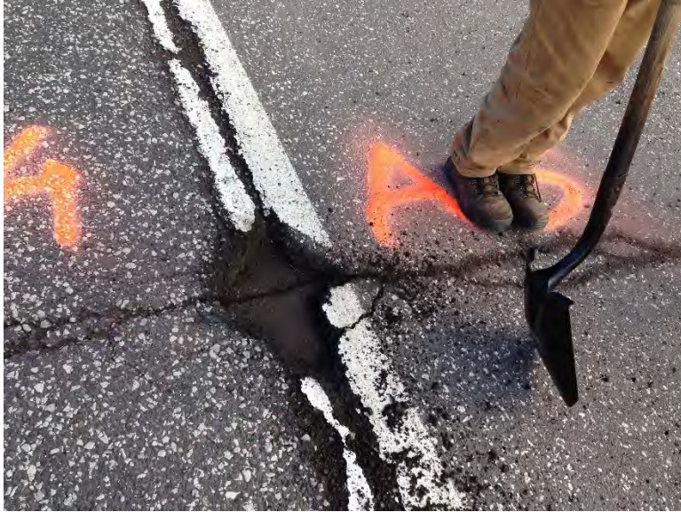
Figure 3.5 Pothole A-5 prior to Patching (After Cleaning).
