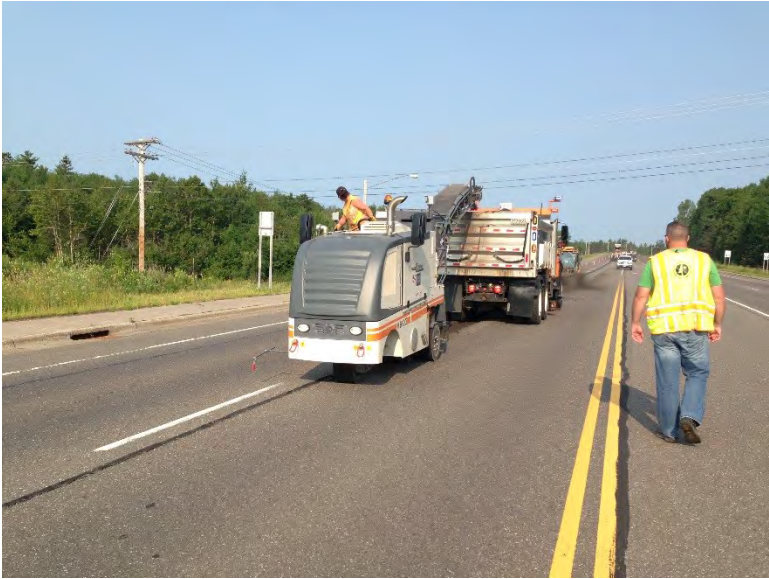
Figure B9: Mill and Fill Step 1.
