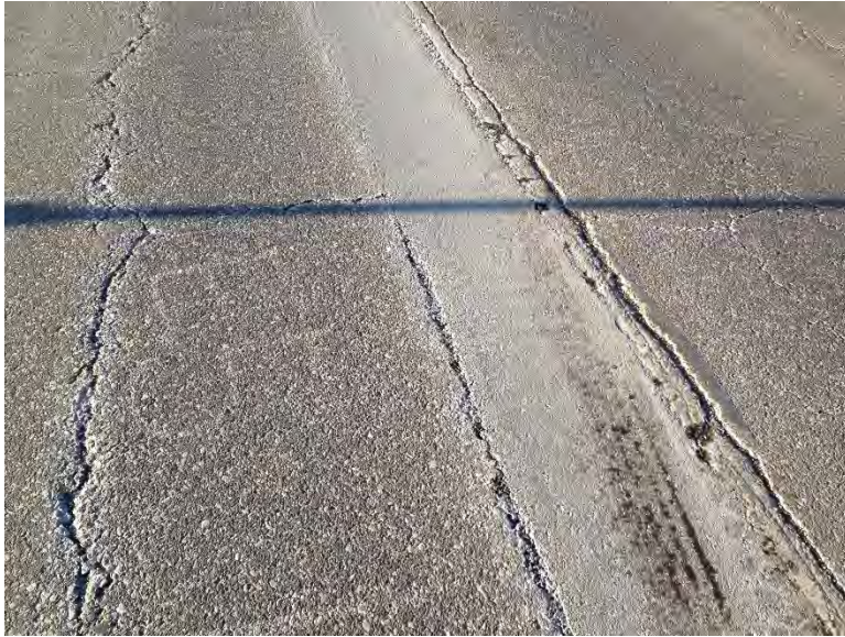
Figure 3.84 Pothole E-5 (119 Days after Installation).
