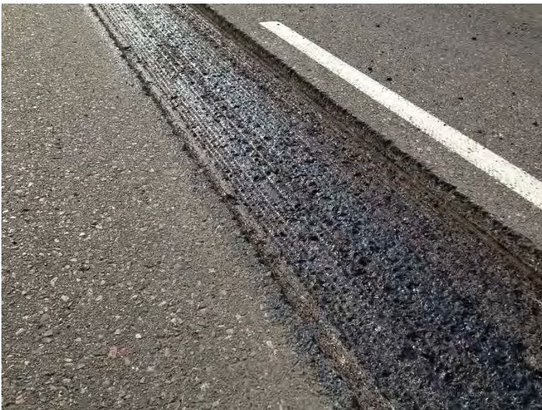
Figure 3.57 Milled Trench.
