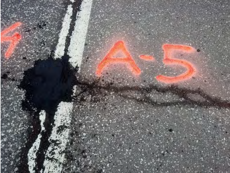
Figure 3.10 Pothole A-5 after Patching.
