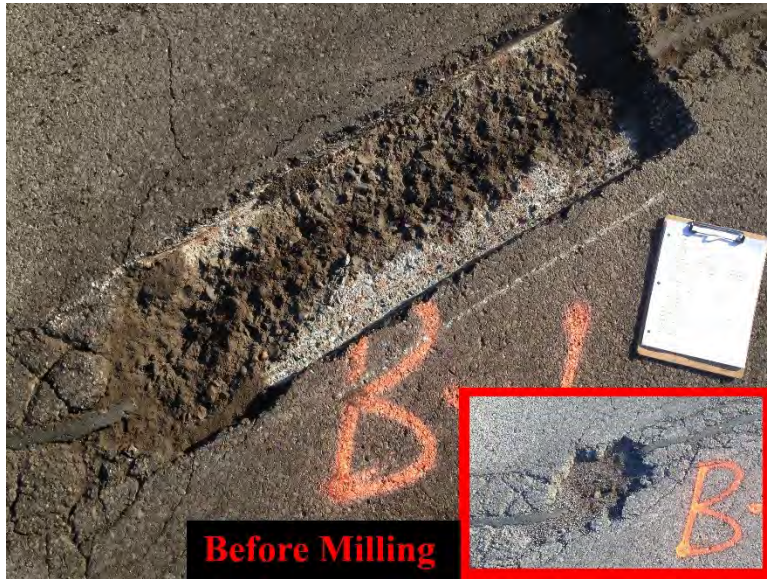
Figure 3.25 Pothole B-1 before and after Milling.
