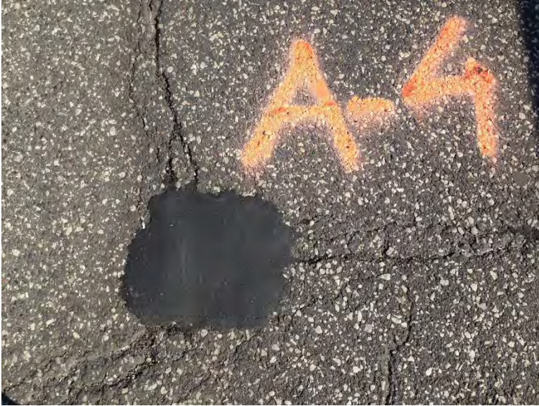
Figure 3.15 Pothole A-4 (3 Days after Patching).
