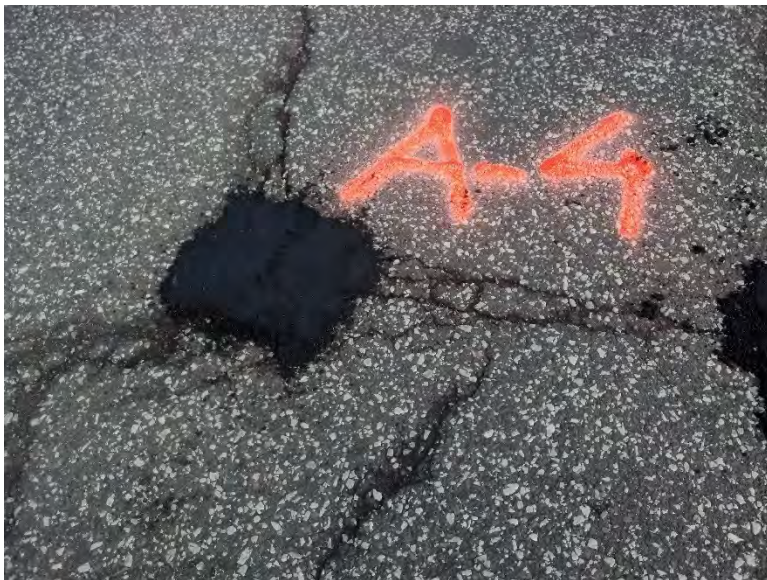
Figure 3.14 Pothole A-4 after Patching.
