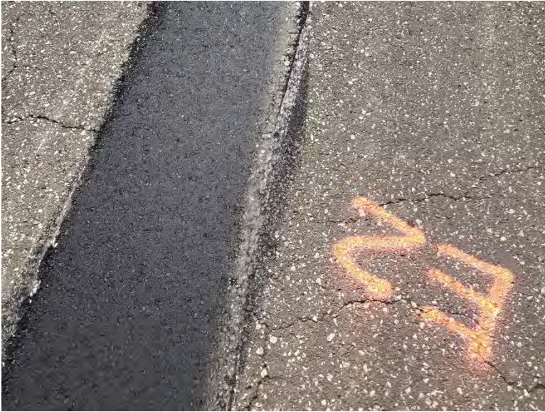
Figure 3.73 Pothole E-2 after Compaction.
