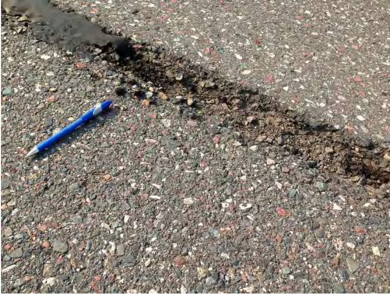
Figure 3.56 Section of Longitudinal Crack with Sealer Missing.
