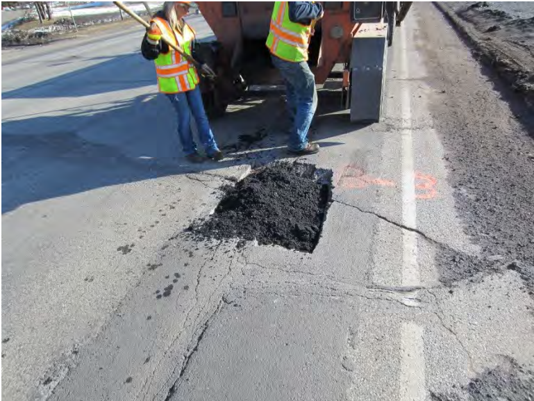
Figure B3: Cold Mix Step 3.
