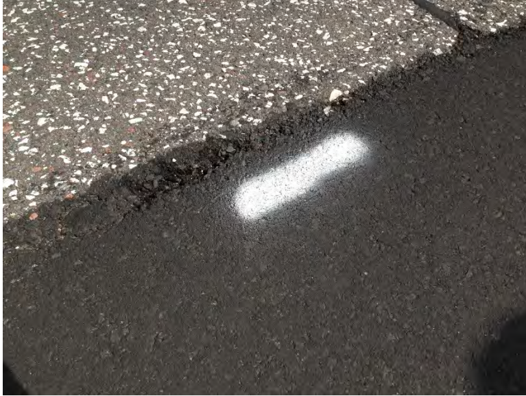
Figure 3.80 Poorly Compacted Interface (28 Days after Patching).
