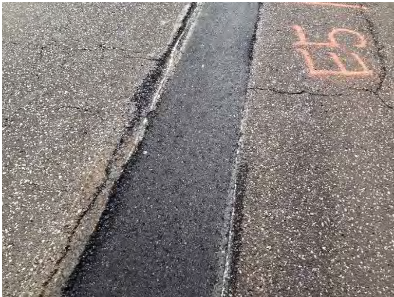
Figure 3.76 Pothole E-5 after Compaction.
