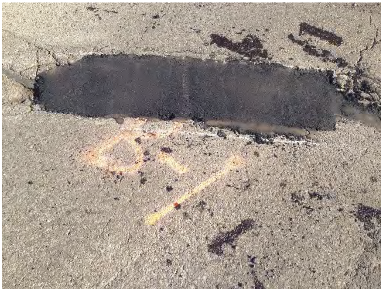
Figure 3.36 Pothole B-1 after Patching.
