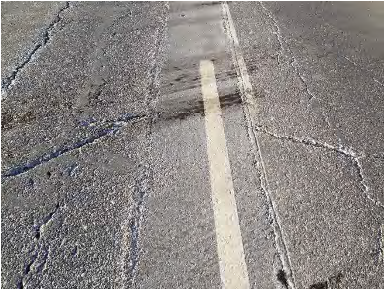
Figure 3.83 Pothole E-4 (119 Days after Installation).
