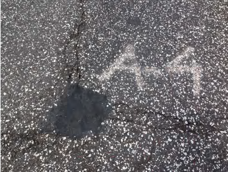
Figure 3.16 Pothole A-4 (149 Days after Patching).
