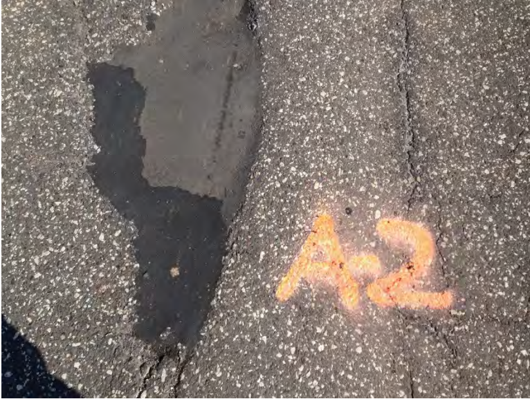
Figure 3.11 Pothole A-2 (3 Days after Patching).
