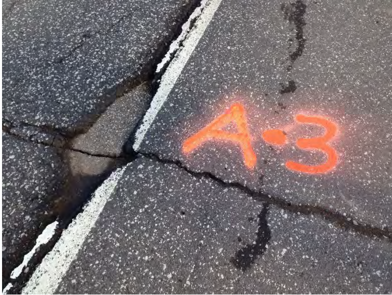
Figure 3.3 Pothole A-3 prior to Patching (After Cleaning).
