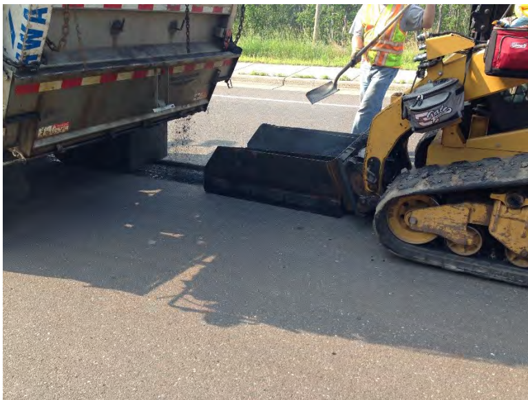
Figure B12: Mill and Fill Step 3.
