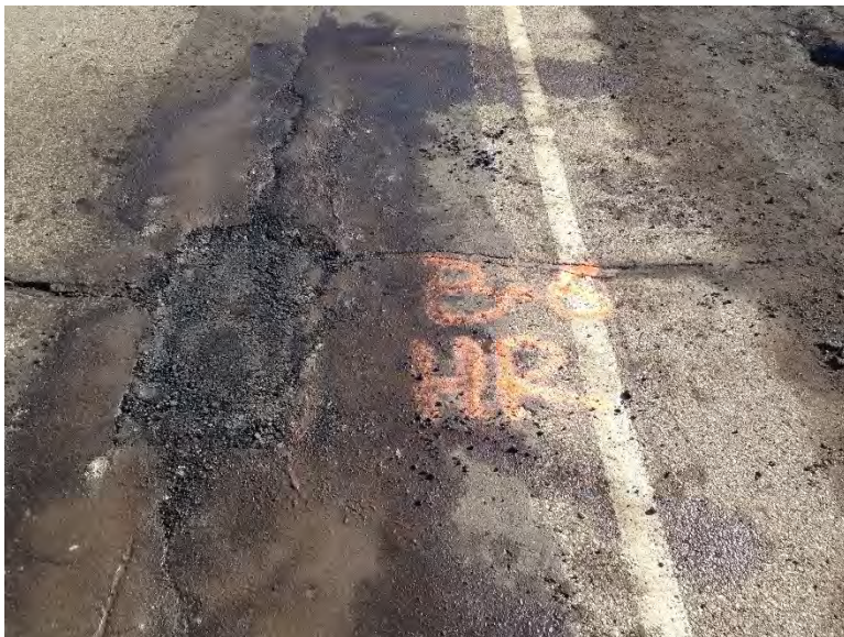
Figure 3.35 Pothole B-6 after Patching.
