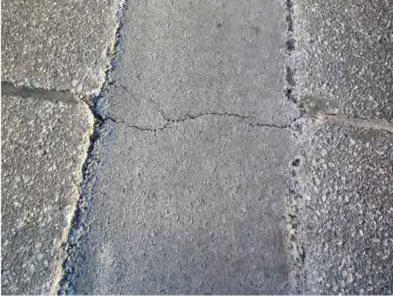
Figure 3.82 Cracking of Pothole E-3 (119 Days after Installation).
