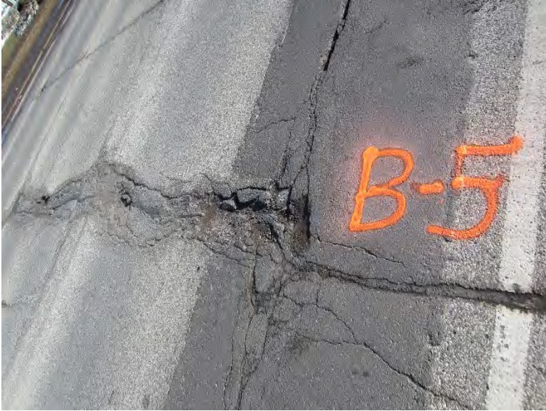
Figure 3.29 Pothole B-5 before Milling.
