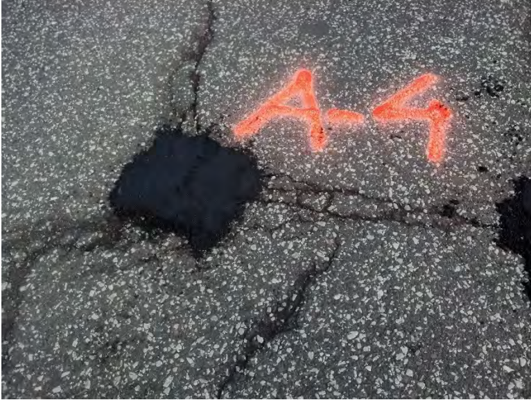
Figure 3.9 Pothole A-4 after Patching.
