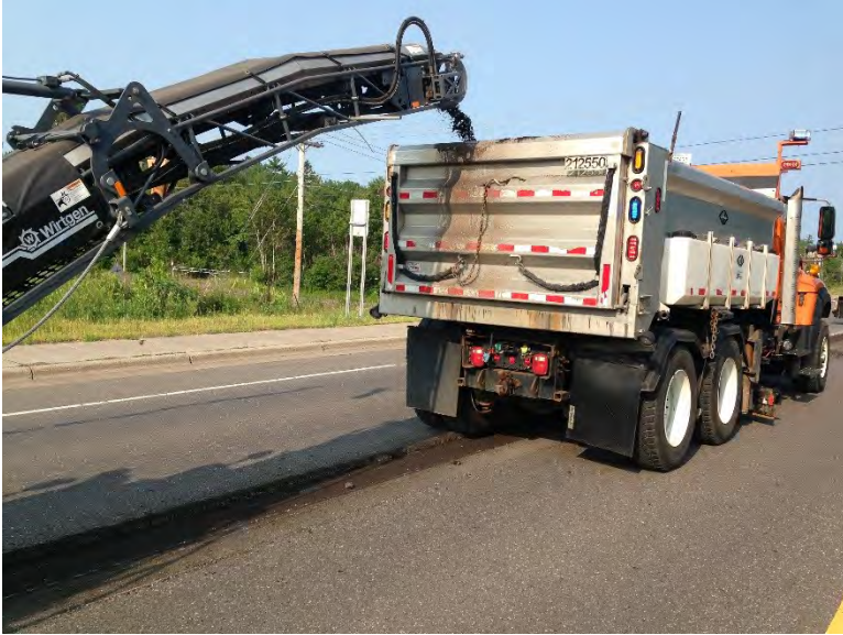
Figure B10: Milled Material is placed in a Truck to be Hauled Away.
