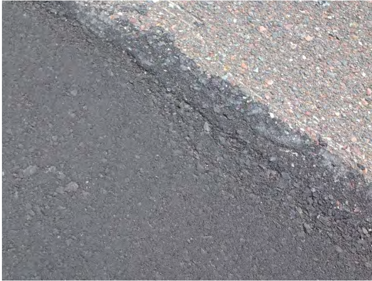
Figure 3.66 Patch Interface (35 Days after Patching).
