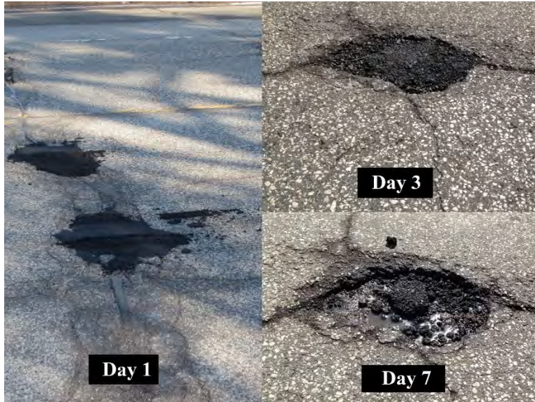
Figure 3.48 Uncompacted Hot Recycled Material in Wheel Path.
