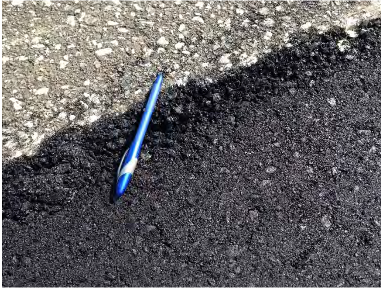
Figure 3.77 Lack of Compaction and Material near Interface of Patch Material and Roadway.
