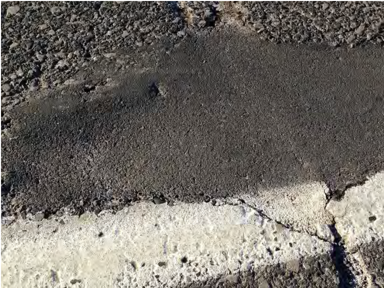
Figure 3.20 Pothole A-5 (240 Days after Installation).
