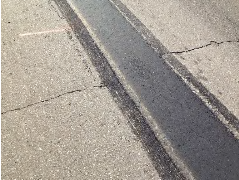
Figure 3.61 Pothole D-3 with Clean Compaction.
