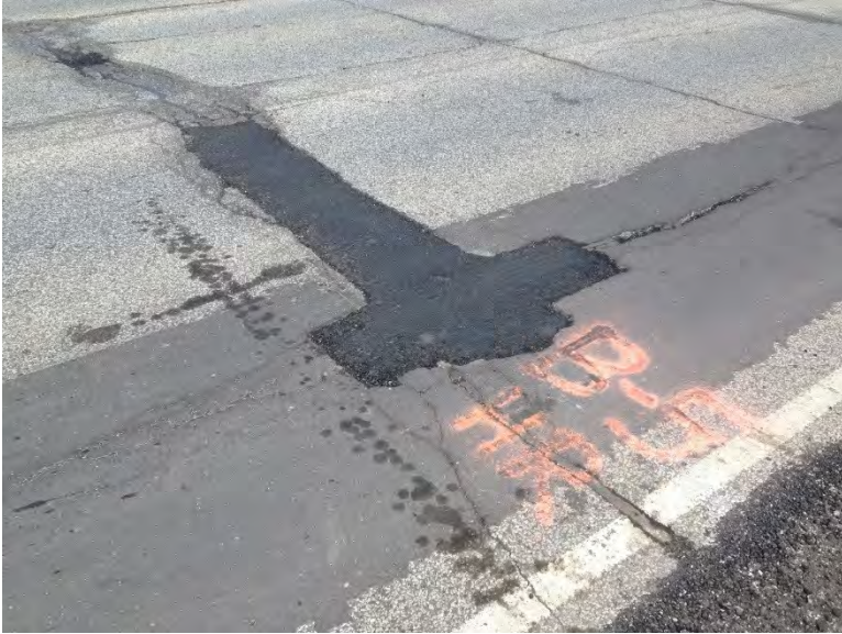
Figure 3.43 Pothole B-5 (3 Days after Patching).
