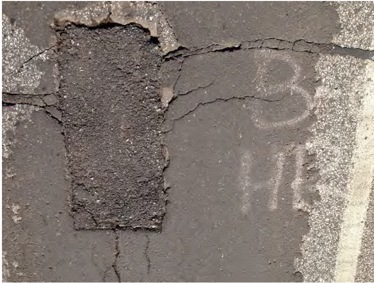
Figure 3.47 Pothole B-6 (146 Days after Patching).
