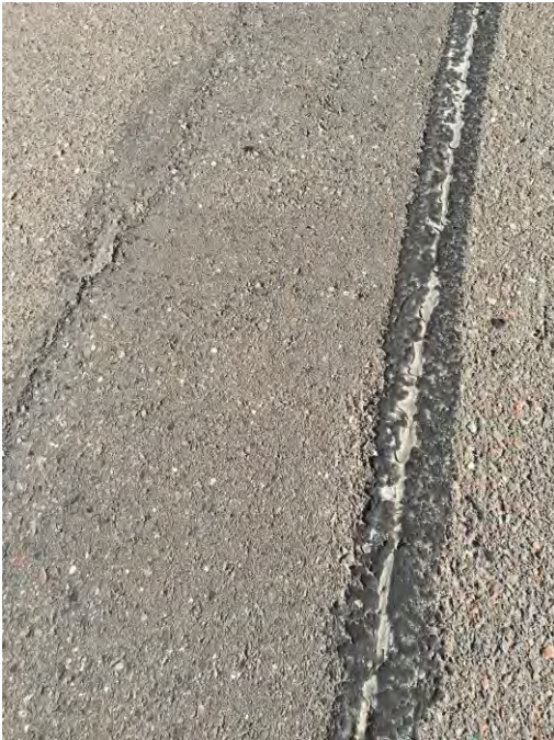
Figure 3.70 Pothole D-2 (426 Days after Patching).
