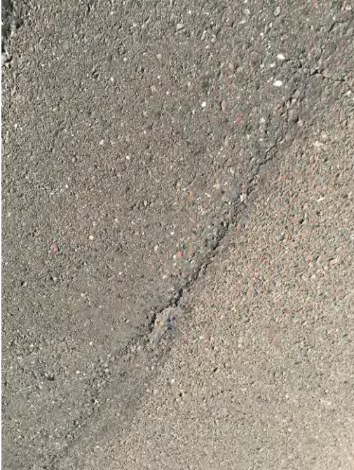
Figure 3.69 Pothole D-1 (446 Days after Installation).
