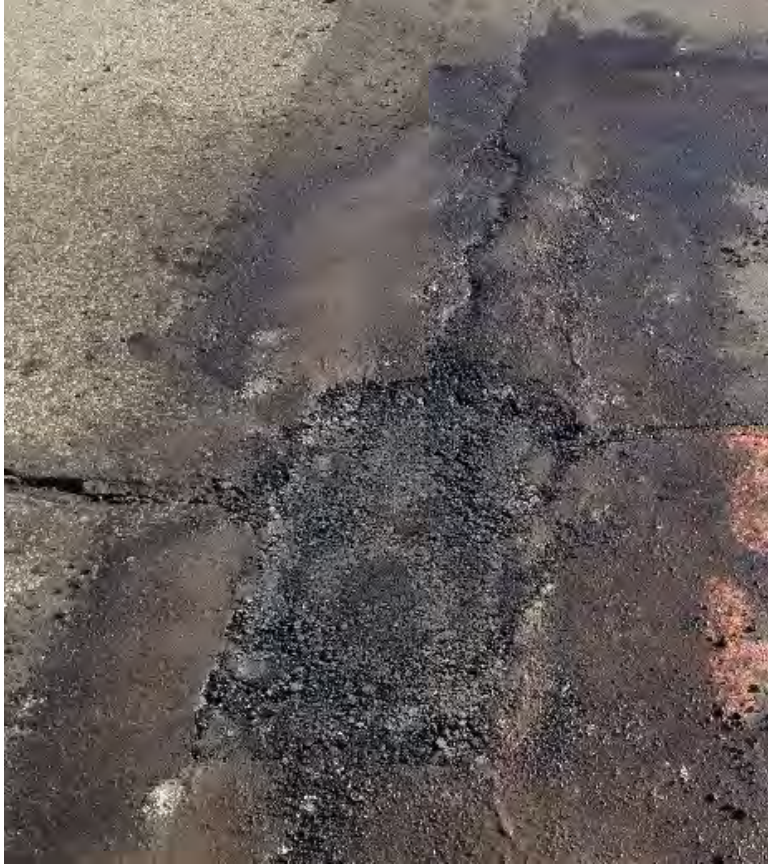
Figure 3.45 Pothole B-6 immediately after Patching.
